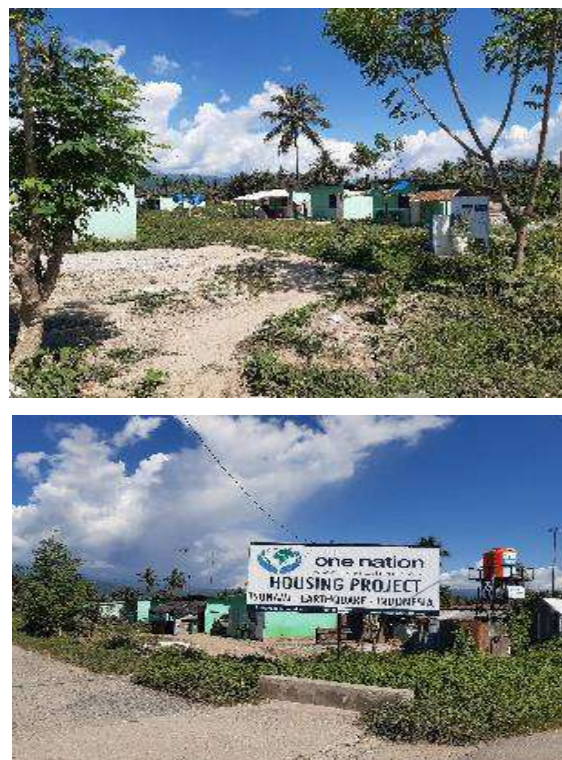
Figure 15. Condition of the Shelter in Dusun III, Langaeso Village
