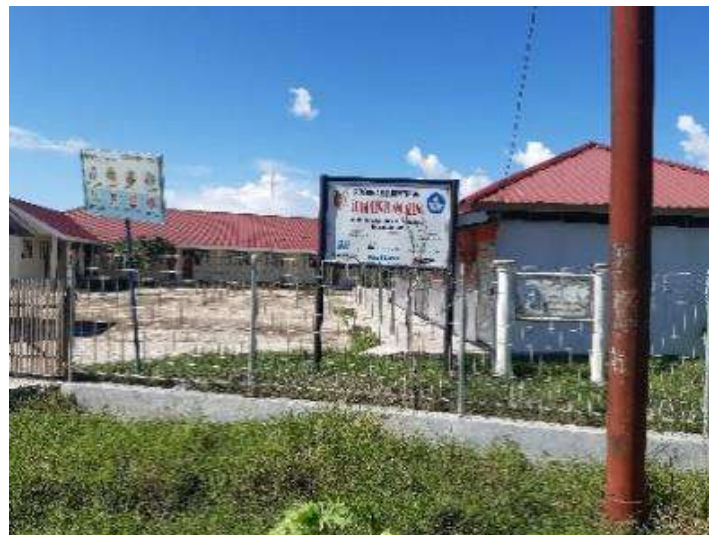
Figure 17. SDN Inpres 2 Langaleso, which was rebuilt with the assistance of an NGO
