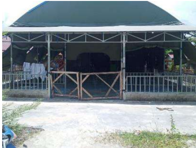
Figure 18. Temporary Mosque in Dusun III, Langaleso Village
